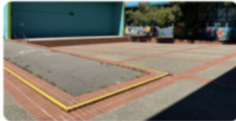
EXISTING SITE PHOTOS
